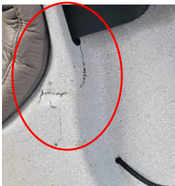
Figure 7-1 (Example of a crack in the cabin floor)
